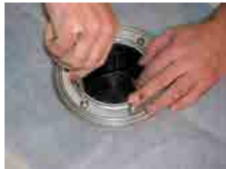
5. Fix the stainless steel ring by screwing
