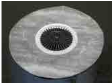
2. Apply prime coat on the raw ceiling
