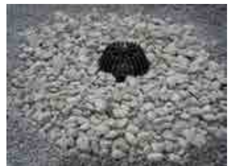
12. Fill with gravel
