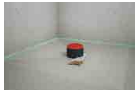
6. After the floor screed is dry, cut the salient nozzle with a saw (or cutting disc).
