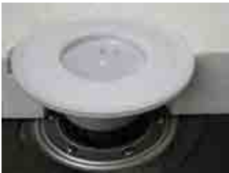
4. Shorten extension with flange (HL85N) and adjust to the height of the thermal insulation, set on the gravel guard (HL180), set the lot cover
