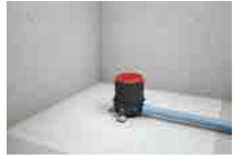
3. Fix the drain body with fixing angles on the floor and connect to the pipe.
