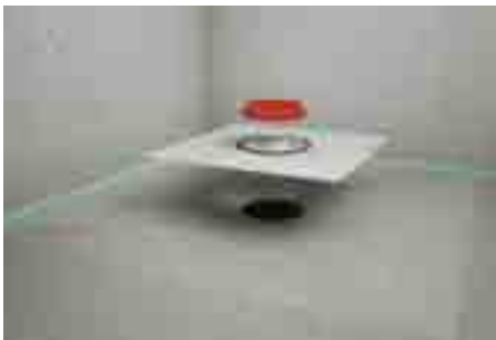
7. Insert the sealing kit, turn the protection cover and insert it again.
