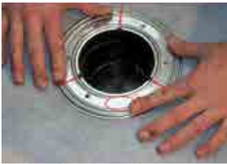
4. Apply the waterproofing membrane
