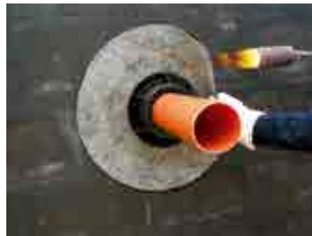
5. Weld the bitumen waterproofing
