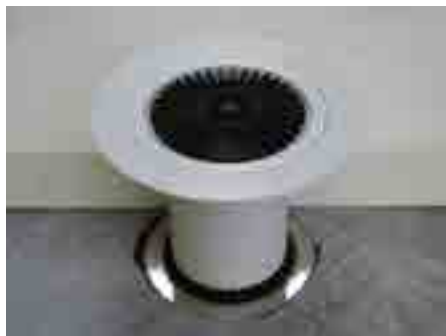
8. Set the thermal insulation plates, adjust the height of the extension by cutting
