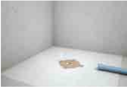
1. Define outlet position, set the stencil in direction to the outlet pipe and mark the holes for the drilling.
