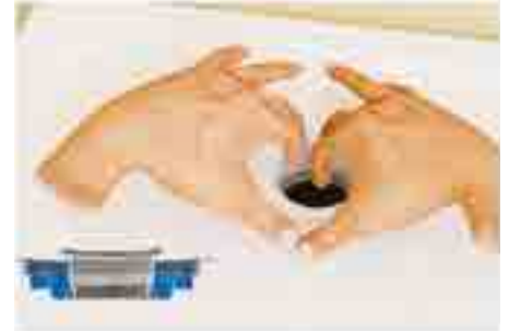
15. Connect flex-element with bottom ring of the counter nut • Dont forget: Leak test • After leak test insert lot cover again
