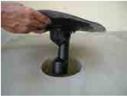
1. Set gully including lot cover into the tap hole
