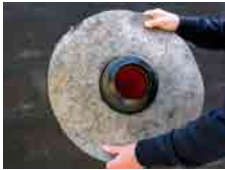
2. Set on bitumen sleeve
