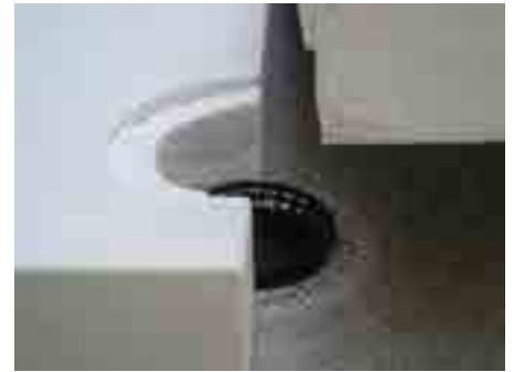
3. Set the fleece, put on the gravel guard (HL180), apply the thermal insulation
