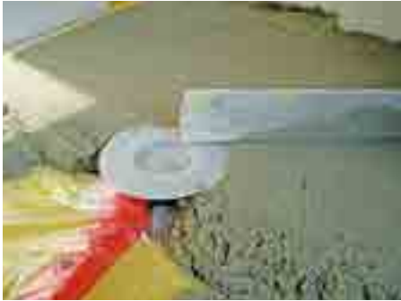
1. Fill in concrete and level to the height of the lid cover
