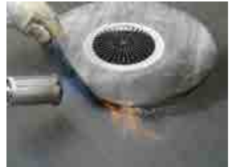
3. Weld the first bitumen layer on the raw ceiling, then weld the bitumen flange of the drain on the bitumen layer
