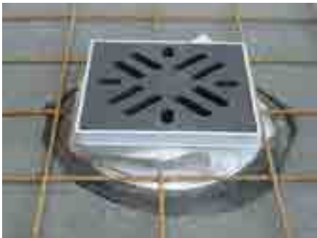
7. Cover the extension with the fleece, lay on the construction steel
