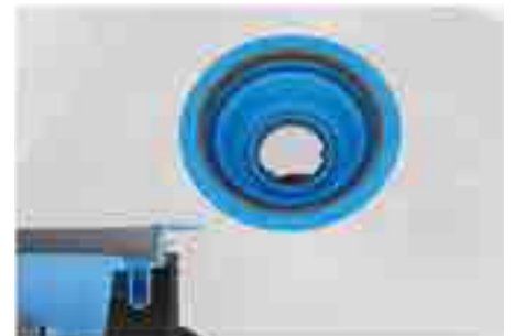
9. Insert sealing kit (flex-element) in the drain body
